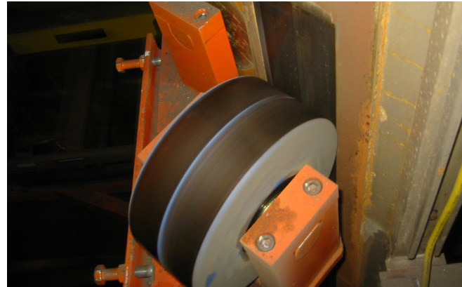
Floor-to-floor elevator guide wheel of NYTEC-HS
